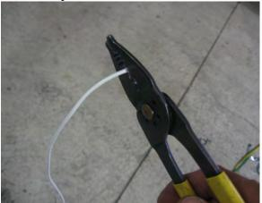
Cut the white ground wire at the front of the trailer leaving it 22" long. Strip the wire and install a ring terminal as previously described.
