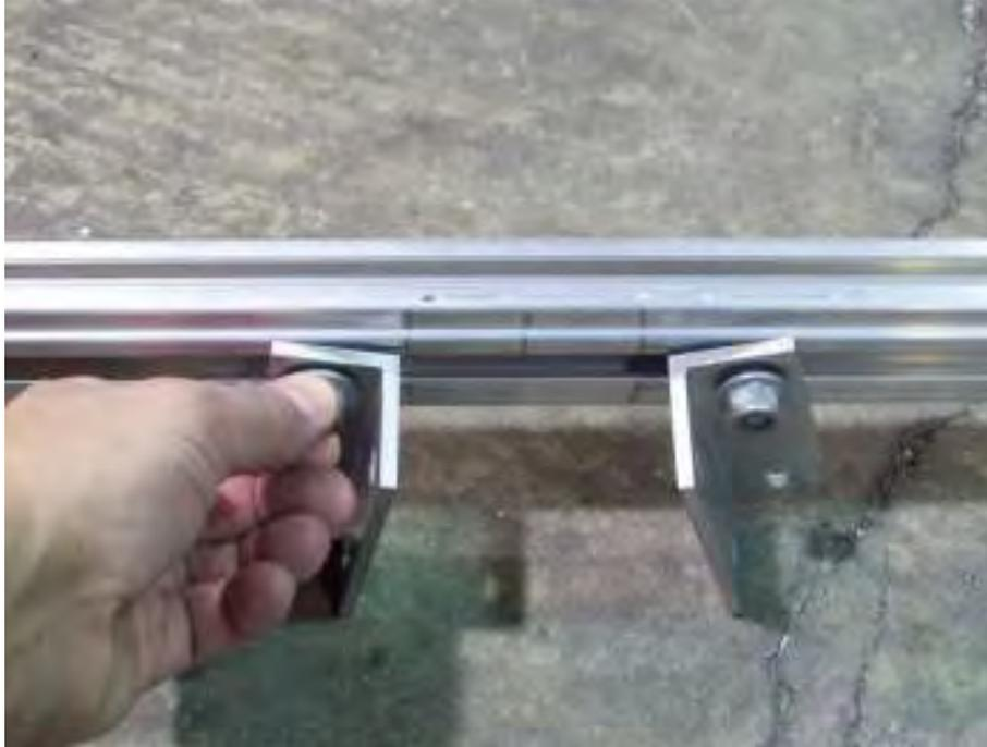
Install the angle brackets on the T-bolts, already in the cross members as shown.
