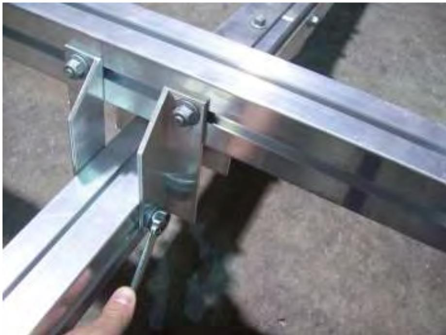
Align angle brackets with pencil marks on the cradle holder. Reinstall nuts and tighten into position.
