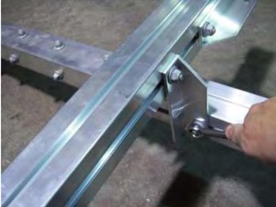
Reinstall nuts and tighten.
