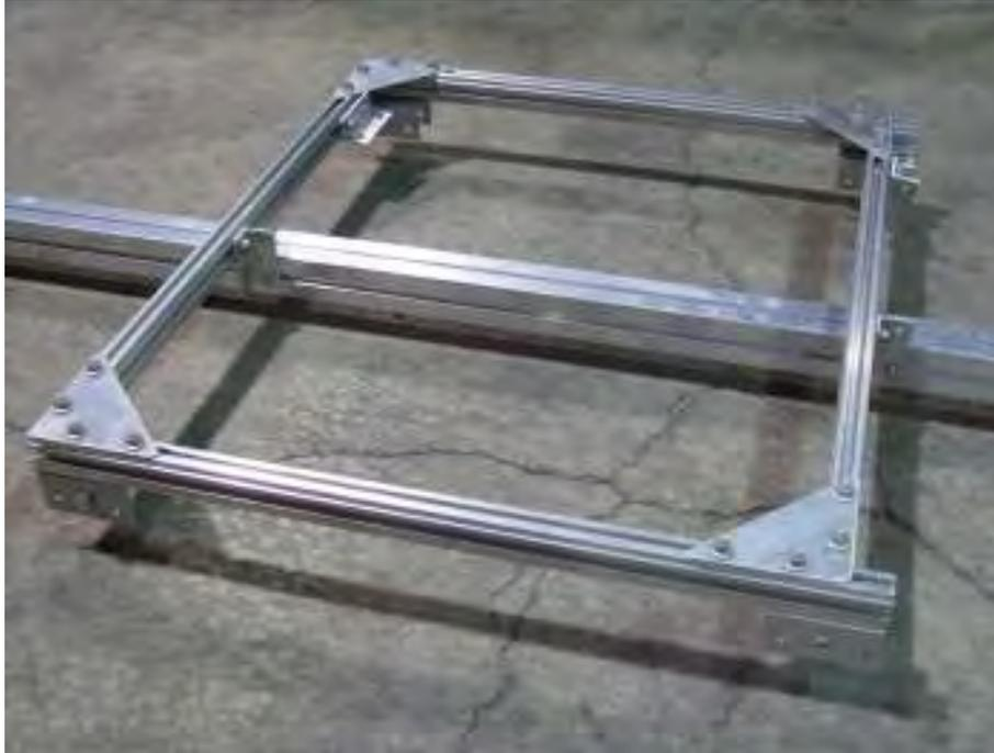
Install angle brackets over top of the T-bolts in the tongue.
