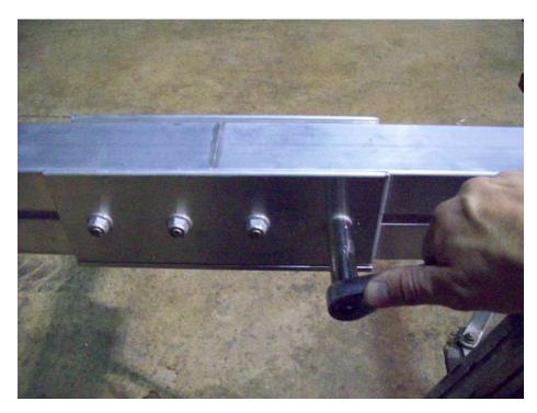
Once plates are in position with no gaps, tighten all nuts.
