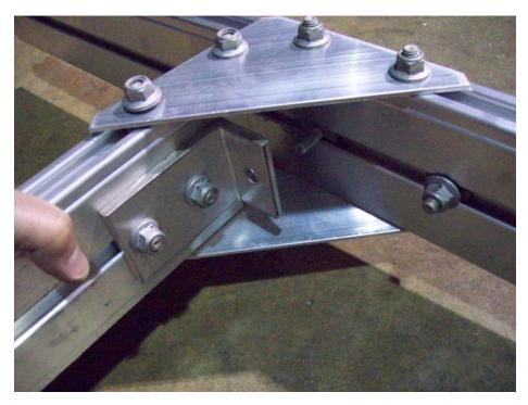
Insert the side rail into the T-bolts on the triangle plate and the cross arm. Once inner angle bracket is over T-bolt, reinstall nut.
