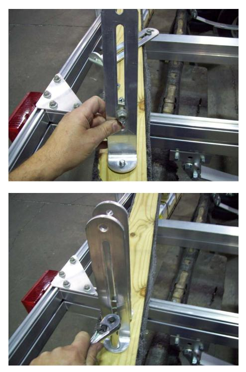
Install slotted brackets on the underside of the 6' padded cradle as shown. Reinstall nuts and lock washers, then tighten nuts. Repeat the process for the other cradles.
