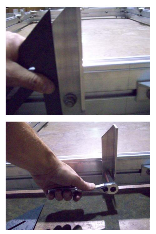
Align back edge of angle with pencil mark on cross arm. Square up angle and tighten. Leave the other angle down at this point.
