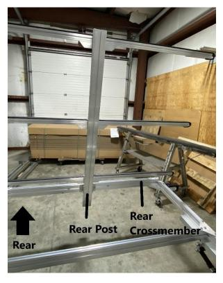
Two people will be necessary to install the rear post. Install the rear post to the (2) center T-bolts as shown. Replace the locknuts but do not fully tighten yet.
