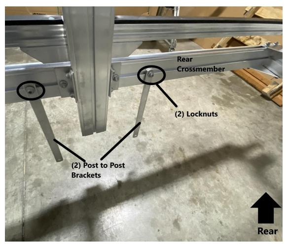
Install (2) post to post brackets using the remaning (2) T-bolts installed in the rear crossmember. Replace the (2) locknuts but do not fully tighten yet.
