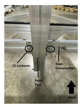
Two people will be necessary to install the front post. Install the front post to the (2) center T-bolts as shown. Replace the locknuts but do not fully tighten yet.
