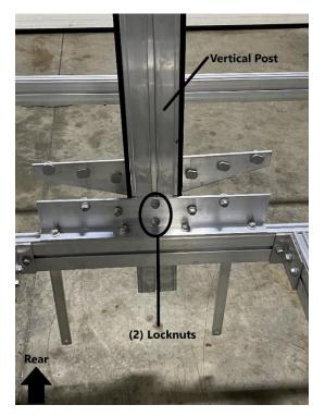
Two people will be necessary to adjust the vertical post. While holding the vertical post, loosen the (2) locknuts and slide the vertical post downward. Tighten the locknuts using a 9/16" wrench.
