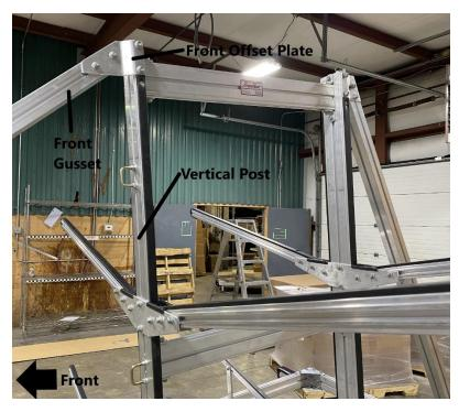
Using a ladder, install the front offset plate and front gusset to the vertical post as shown. Tighten the locknuts using a 9/16" wrench.
