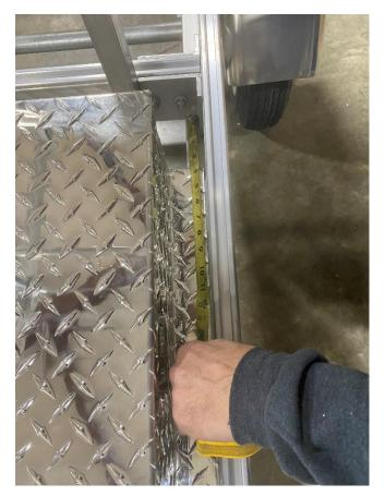
Use measuring tape to confirm that the storage box is centered.
