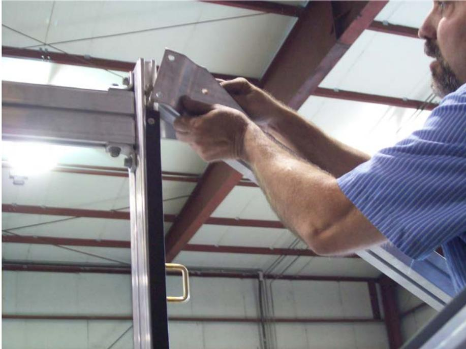
Install the right side top offset attaching plate.
