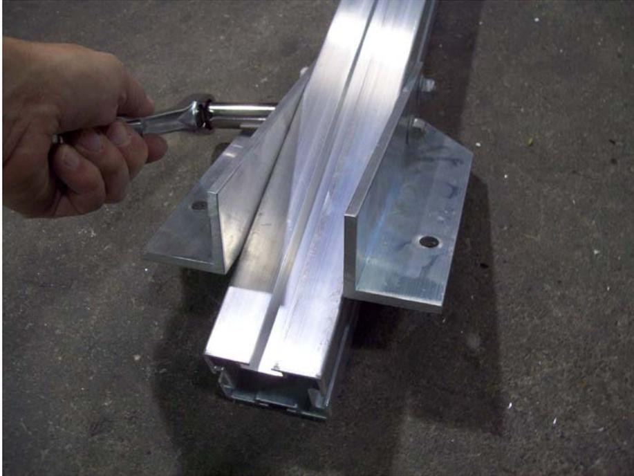
Install both of the bottom attaching angles to the gusset. Slide both angle plates about 2- 3” up on the gusset and snug the nuts.
