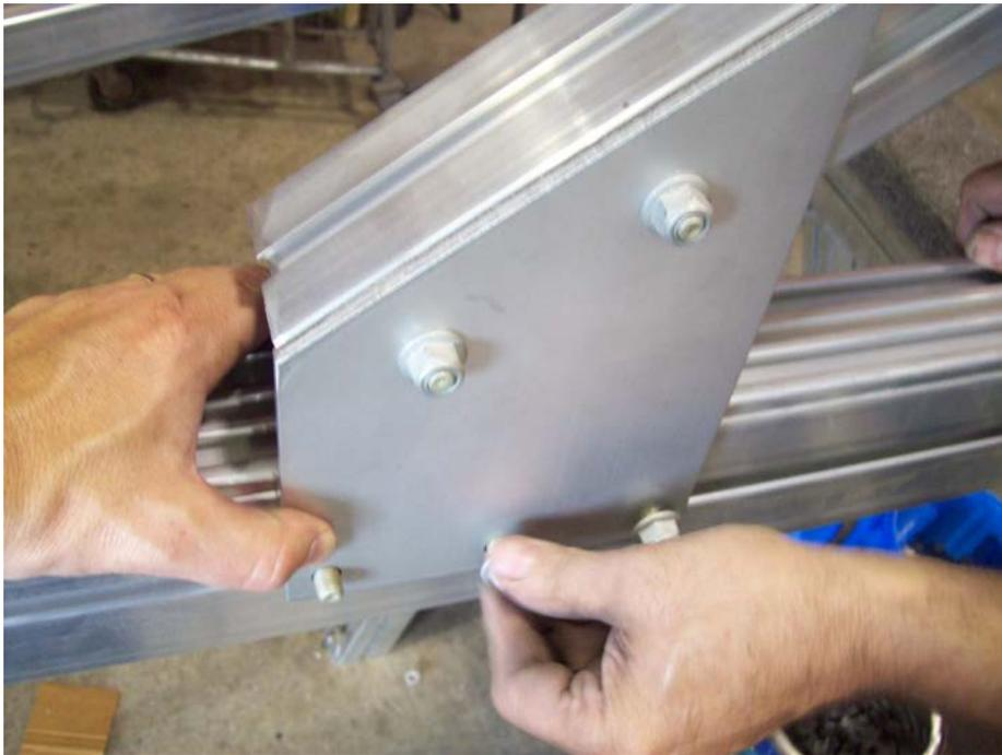
Install the bottom attaching plate onto the three T-bolts on the tongue section. Reinstall nuts but don't tighten yet.
