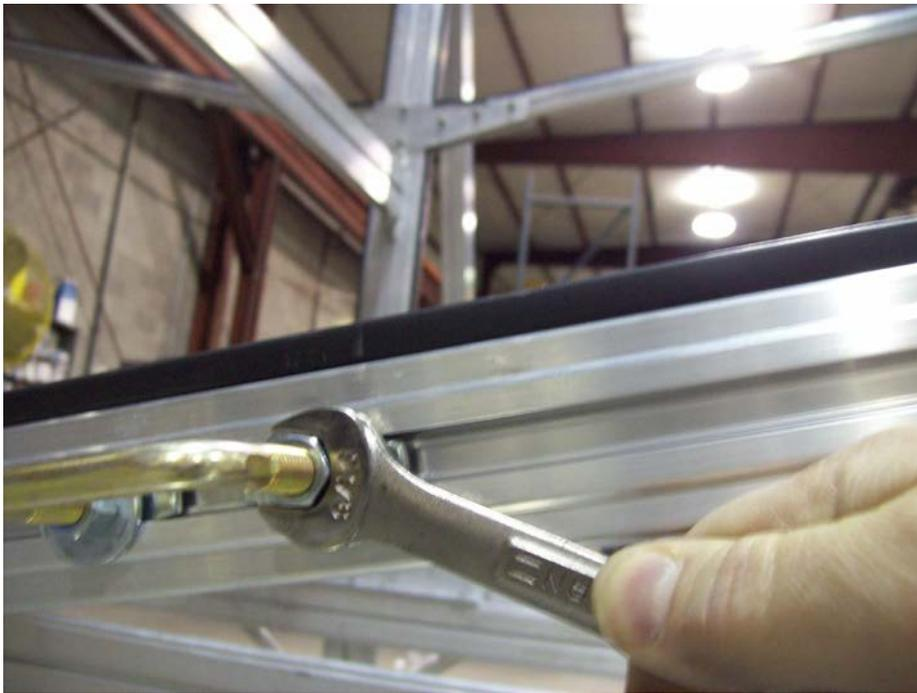
On the bottom cross bars, insert a web strap clip facing out on each arm. Position the web strap clip in the center of the arm and tighten.
