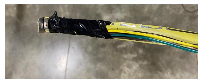
Use electrical tape to attach 4 wires (2 brown, 1 green, 1 yellow) to the end of a tape measure. <u>Do not tape the white ground wire.</u> The white ground wire will stay at the front of the tongue section.
